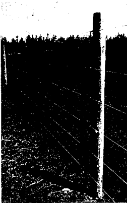
Photo 1 (above) A 6 plain wire electrified fence 1.6 metres high.
