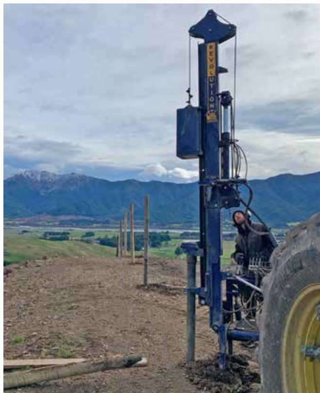
New deer fencing is going in at Wye Hills.
