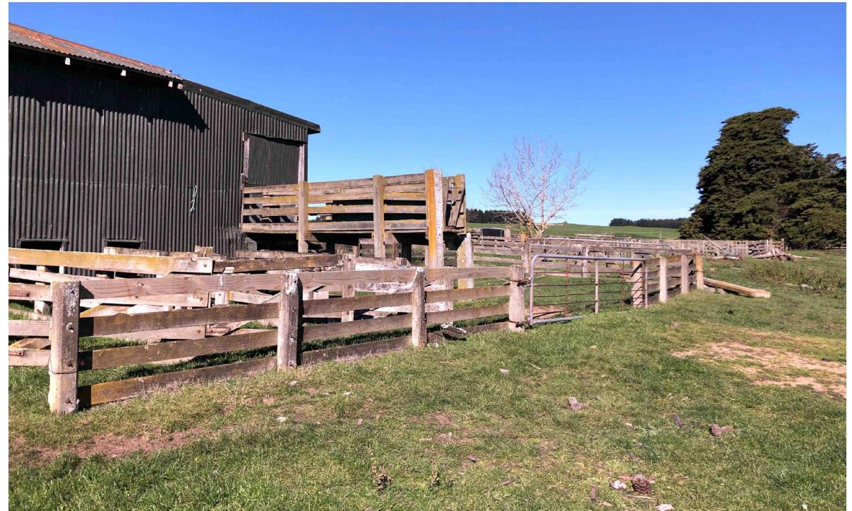
Shed and yards, showing low slope.
