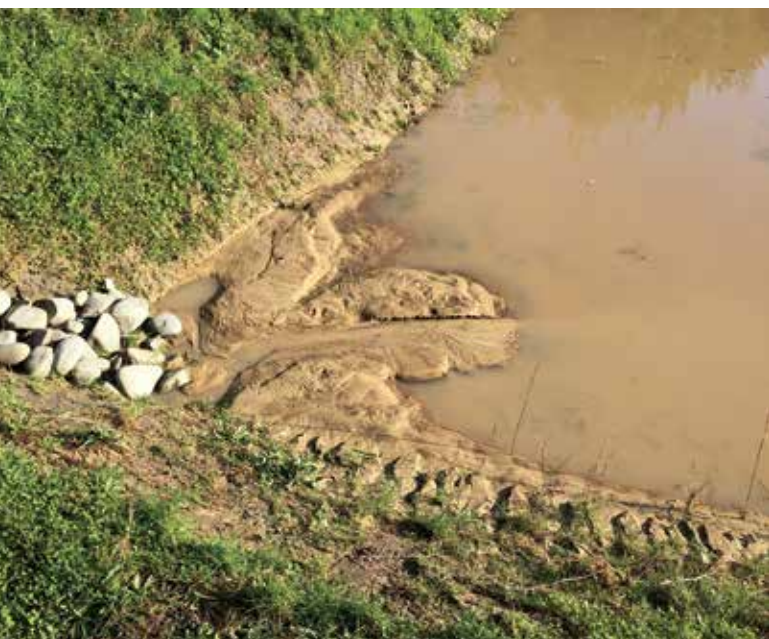
Downstream detainment bunds can do a great job of preventing run-off sediment from contaminating waterways
